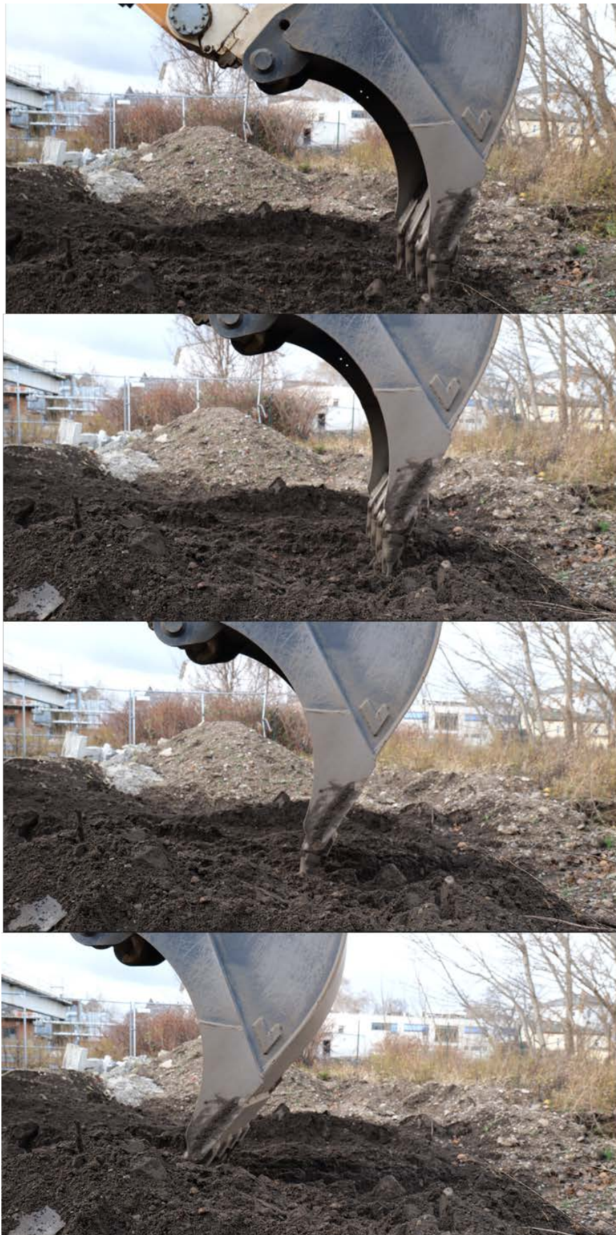
Figure 37: Finish grading: The linear movement of the bucket tip is easily controlled by the operator with the help of the height indicators at the bottom of the arm.
